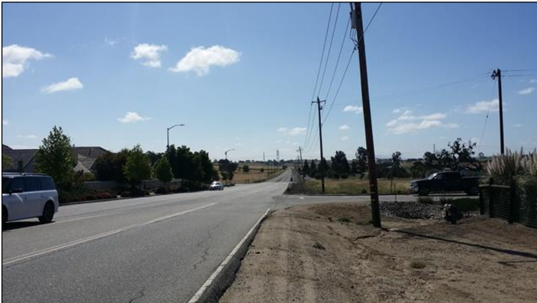
Photo 2: View facing east on Creston Road toward the eastern portion of the project. Dense housing on the north side of Creston Road, intermittent space on the south side.
